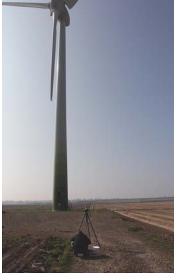
Figure 4. On-site test setup
